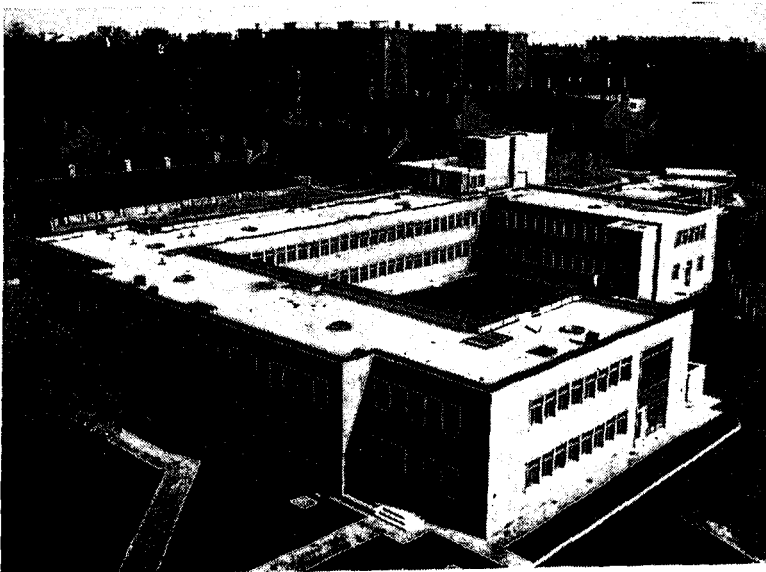
A General View of the Health Centre.
